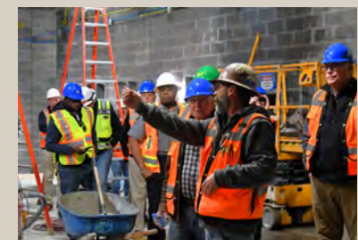
Officials receive update on construction of new detention center, slated for completion in January 2027.
